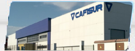
Industrial boiler company 16,000 m 2 | Oñate - Spain
